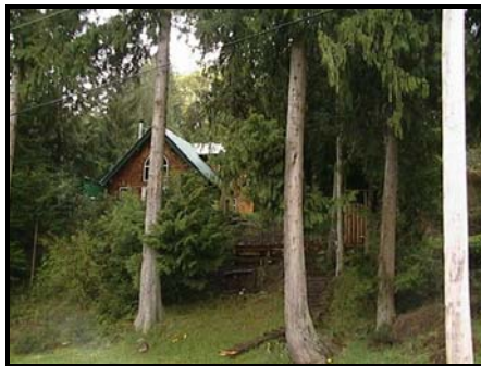
Figure 10: A Wildland Interface Residence. Source: Dave Enfield Fire Chief, Saltspring Island Fire Department.
